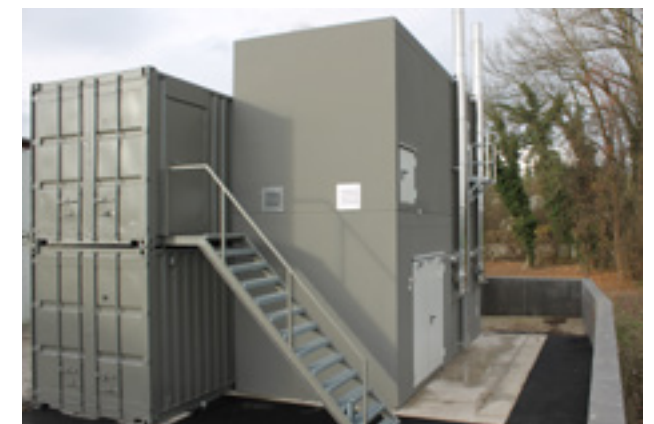
Doppelstock-Heizcontainer 2 x 90 kW Pellets, Industrie
